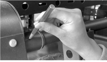
1. With the gate closed and both locking pins in place to secure the gate shut, mark the center of the locking pin hole through the collar as shown.
